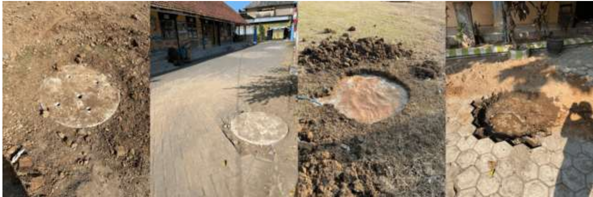
Figure 2. Rainwater infiltration wells installed
